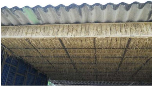
Fig : Roofing panel prepared from paddy straw
