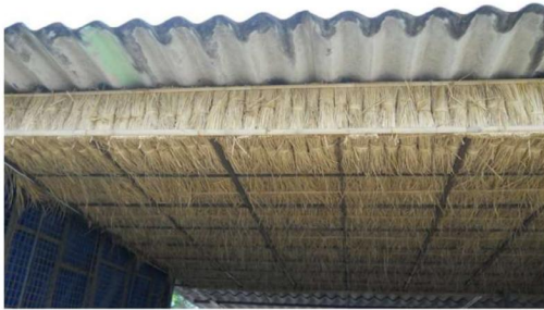
Fig : Roofing panel prepared from paddy straw
